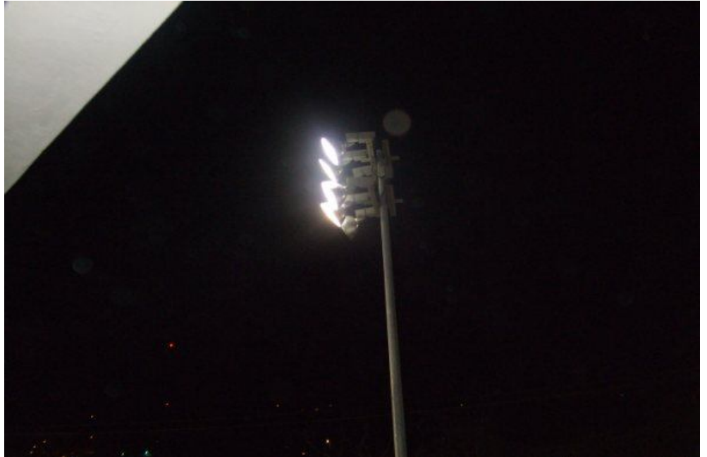
Tobago - Shaw Part Public Tennis Courts – 40' Pole with 6 x SLS1500w luminaries.
